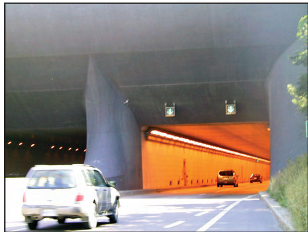
Figure 9 – Thorold Tunnel Lane Control Signs
