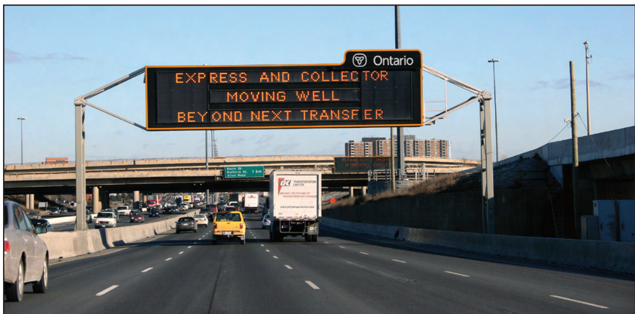
Figure 12 – MTO Overhead Gantry-Mounted DMS
