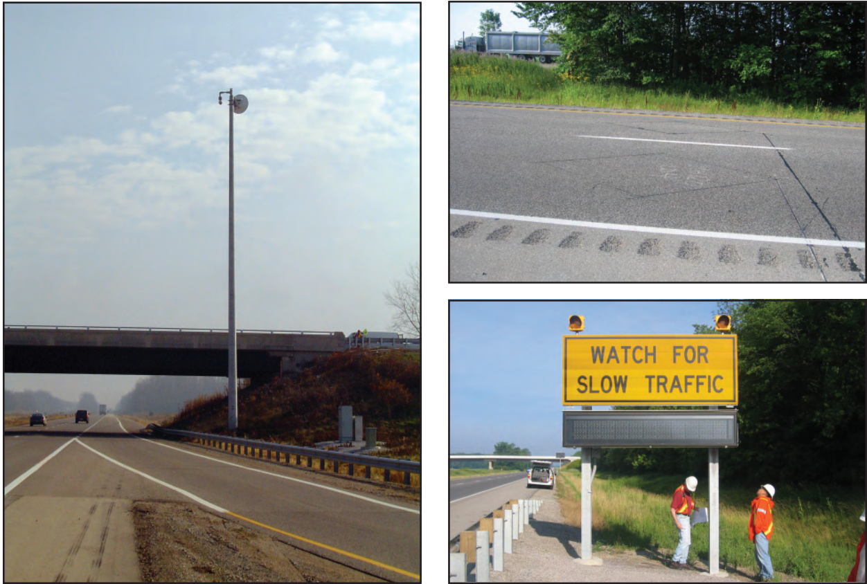
Figure 15 – Typical Elements of a Queue Warning System
