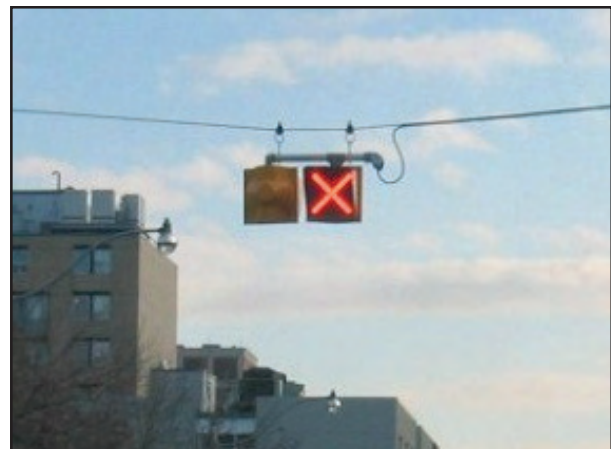
Figure 10 – Jarvis Street Lane Control Signs
