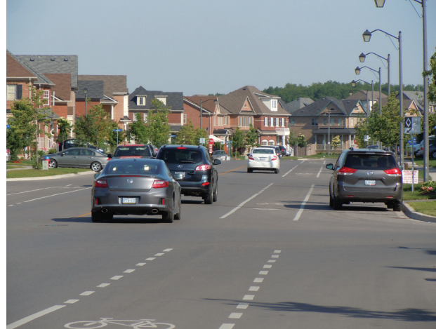
Figure 2.5 – Conventional Bicycle Lane, Milton Trails
