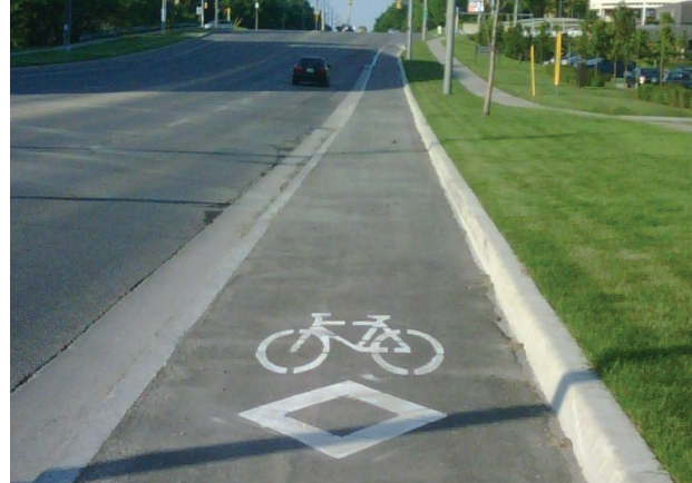
Figure 8.3 – Well Maintained Bicycle Facility
