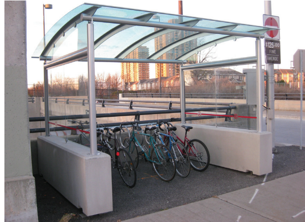
Figure 7.3 – Sheltered Bicycle Parking
