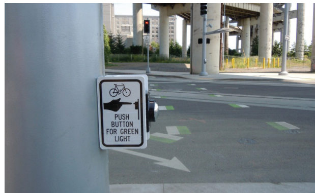
Figure 5.45 - Example of Cyclist Pushbutton
