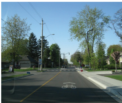
Shared Roadway with Sharrows
